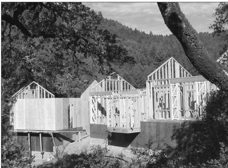
New restroom building (left) and office building (right) under construction
